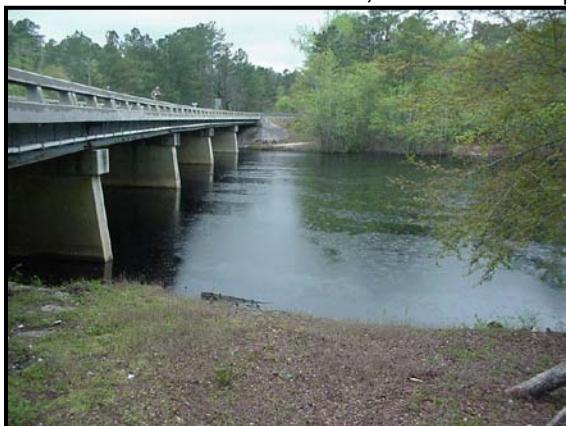
B210- Black River at Hwy 210 bridge
