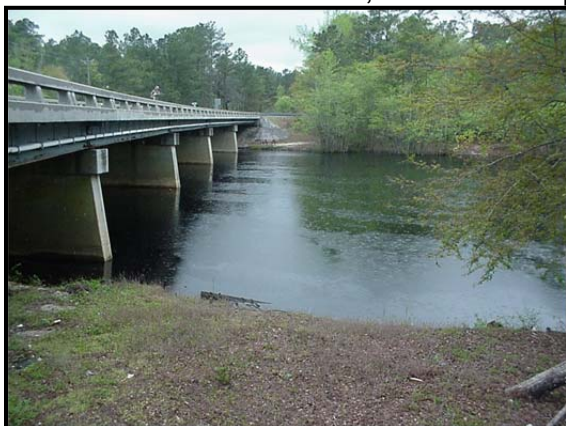
B210- Black River at Hwy 210 bridge
