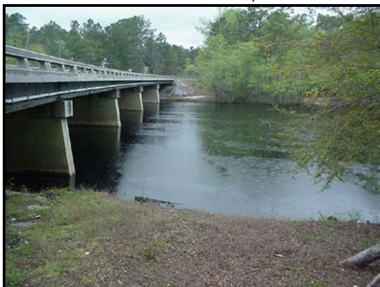
B210- Black River at Hwy 210 bridge
